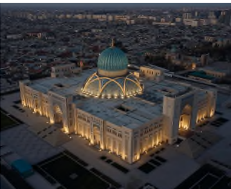
The Center for Islamic Civilization in Uzbekistan. Tashkent
